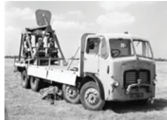
Trial 3 seat ejection for Vulcan V Bomber. (Chalgrove)
